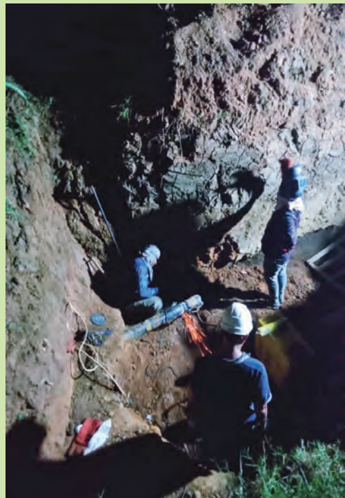
4 inch steel pipeline works for maintenance, flushing 2
