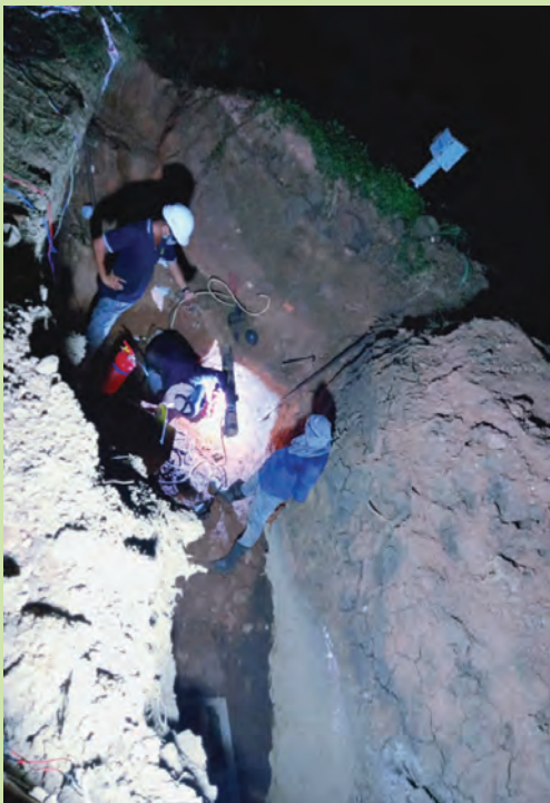
4 inch steel pipeline works for maintenance, flushing 1
